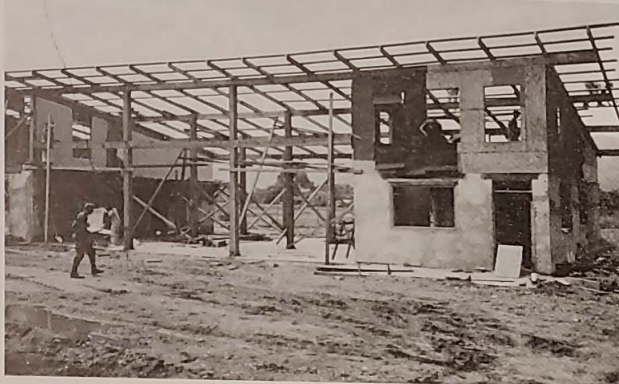
ABOVE: A Honduran Fire Station - BEFORE the 507th Civil Engineers.
